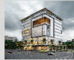
SSBC JKD ELEVATE (Commercial) Gopalpura Bypass
